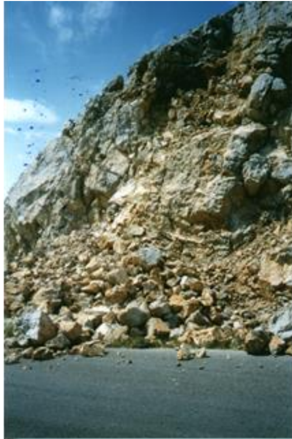
Figure 20- Landslide caused by the 1999 strong earthquake uphill Aspropyrgos town, west side of Attica Region (from Pavlides et al., 2002).
