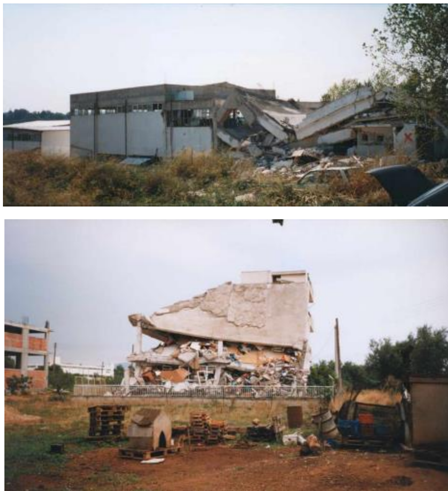
Figure 19- Collapse of a factory building (top) and of residential building (bottom) in the west side of Attica Region resulting from the 1999 strong earthquake (from Papadopoulos, 2000).
